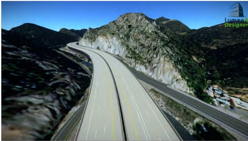
East Portal – Looking West (Figure 4)
